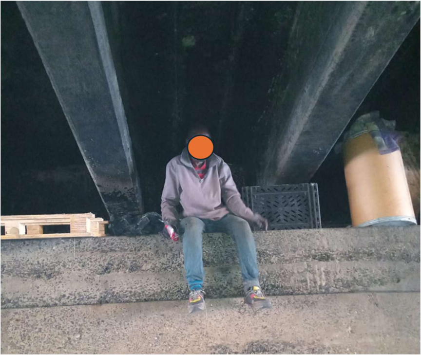
A male was found under the canal bridge where he made himself a home. Nobody was aware until he started making fire under the bridge resulting in the patrol officers removing him out of the area.
